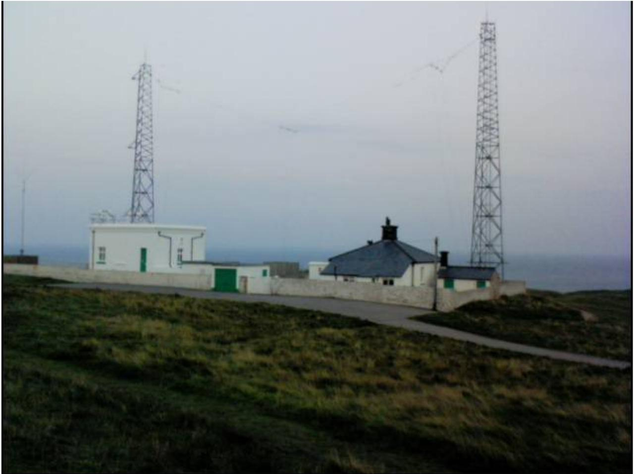
Located on the cliff edge a short distance from the lighthouse, the fog signal is the white square building. The fog signal is a nautaphone which is an electronic device directional to the sea which gives two blasts every ninety seconds. This pattern is again unique to Flamborough and aids navigation and to locate position.
